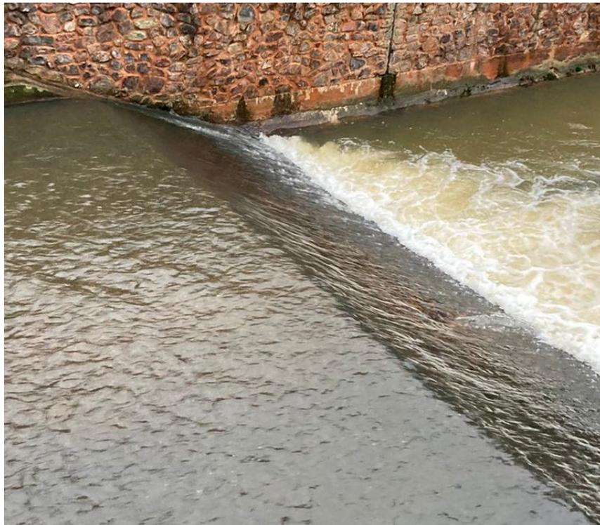
*Figure 7 Sloping weir immediately downstream of the ford*
