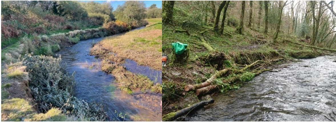
Figure 13: In river wood installation examples. Left: brush and willow stakes added to the riverbank to reduce bank erosion, slow flows and trap sediment. Right: large woody debris added to the river bank to deflect flows and aid in bank protection. Source: WRT
